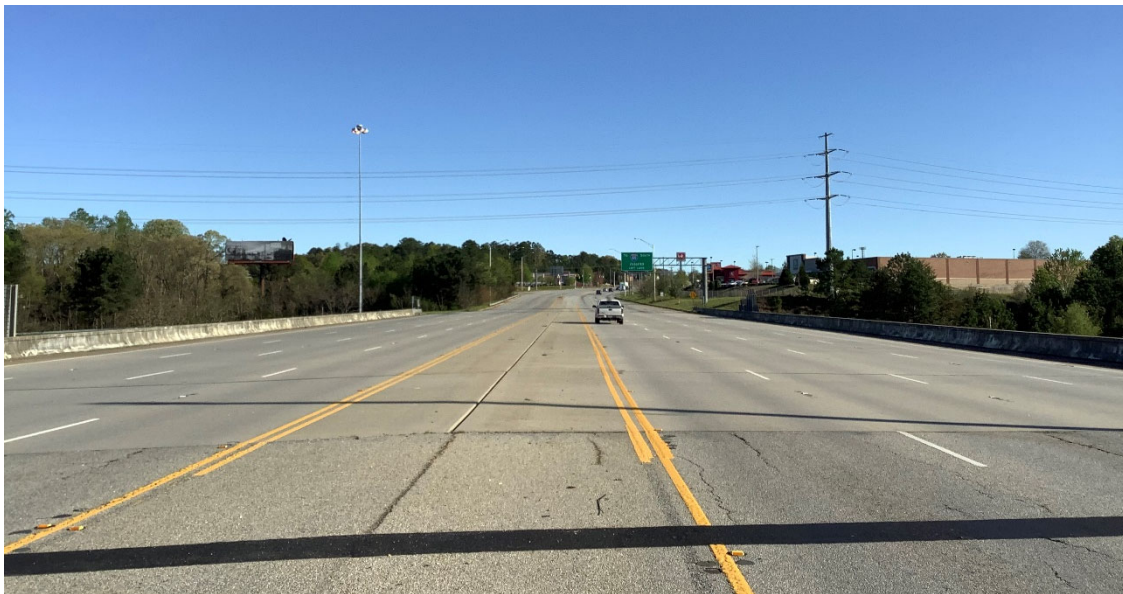
Example: Approach View of a Bridge Superstructure Separated by an Open Longitudinal Deck Joint with No Physical Separation (i.e. Barrier, Raised Median, Etc.)
