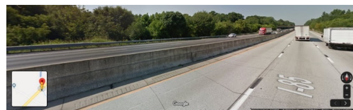
04016 (Anderson) – '3' - Closed Median (non-mountable barriers), culvert beneath, barrier between
