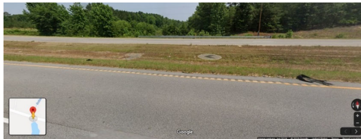
00599 (Chesterfield) – '1' - Open Median, culvert beneath both bounds with grass median between
