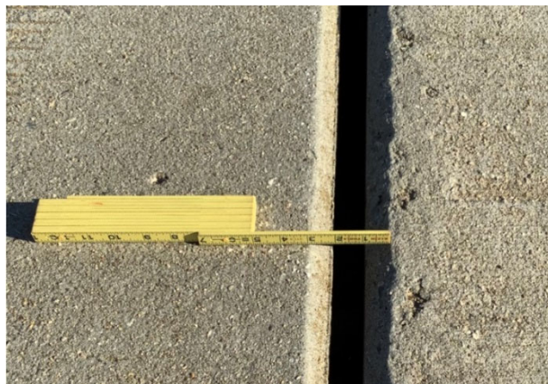
Example: Looking Down at a 1" Open Longitudinal Deck Joint
