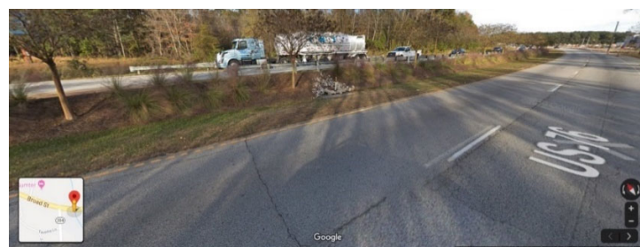
01228 (Sumter) – '2' - Closed Median (no barriers), culvert beneath both bounds with grass/tree median
