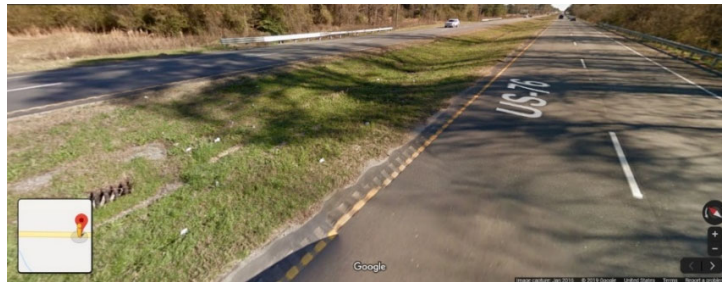
02350 (Florence) – '0' - No Median, culvert beneath both bounds with grass median between
